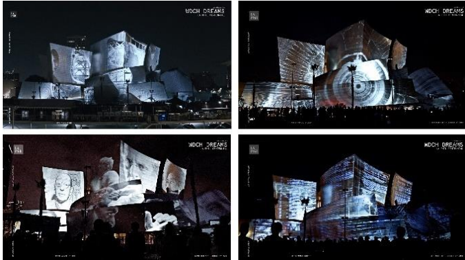
Figure 3. 158: WDCH, Public art installations projected onto the building's surfaces (Url 26).
