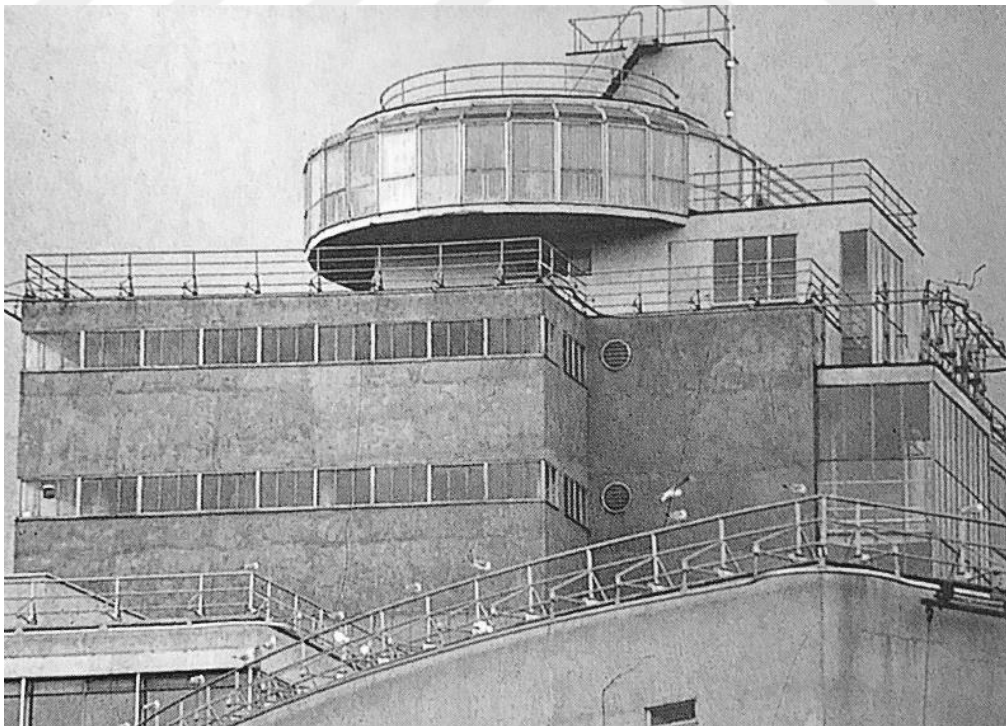
Figure 2. 33: Van Nelle Factory, circular roof structure (Hertzberger, 2005, g. 218).
