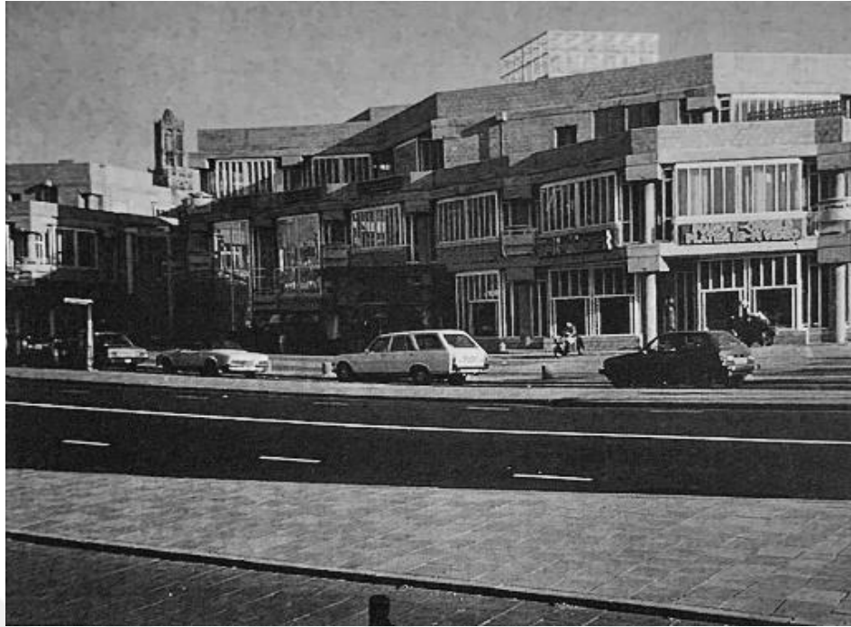
Figure 3. 29: VMC, a photograph of the building from the outside (Hertzberger, 2005, p. 136).
