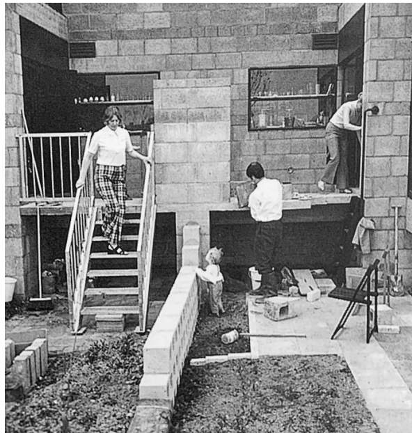
Figure 3. 11: Diagoon Dwellings, a photograph of the outdoor conversion into living space (Stegeman, as cited in LSA, p. 159).
