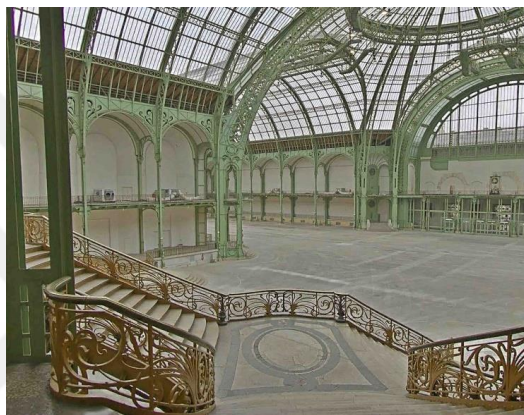
Figure 2. 19: Grand Palais, wide openings created with steel structure (Google Earth Pro).
