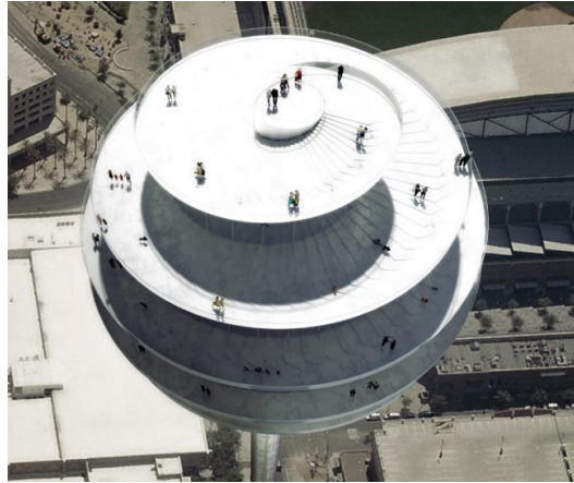
Figure 3. 130: POT, The spiral form of the building (Url 19).
