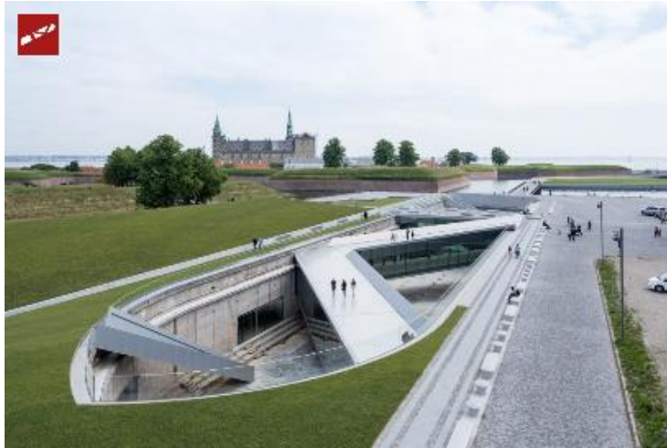
Figure 3. 136: DMM, a photograph of the general view (Url 20).
