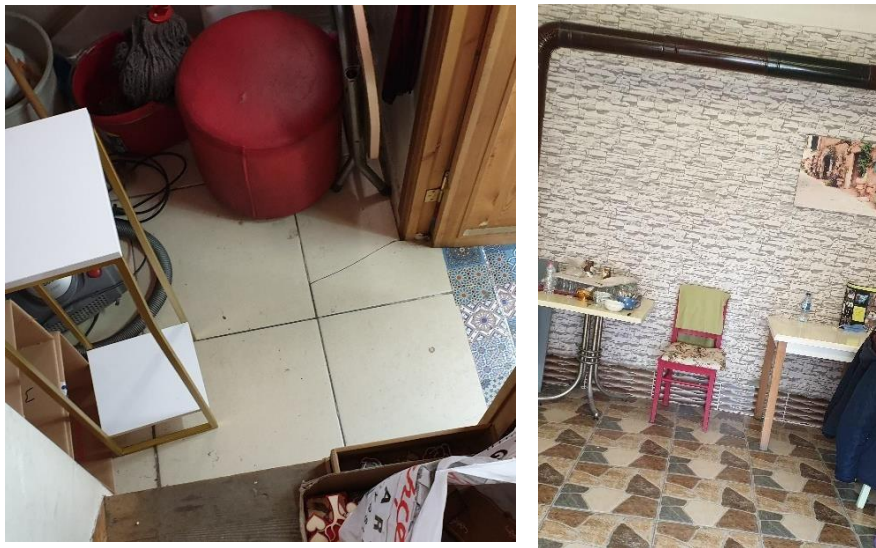
Figure 3.30: Examples of material variety at the interiors of the buildings on Dutlu Street (Çakıroğlu, 2021)
