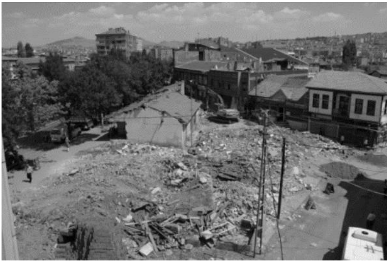
Figure 3.13: View from M. A. Ersoy Street in 2006 showing the collapsed buildings due to negligence in the study area (Arslan, 2012)
