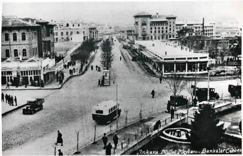
Figure 3.9: View of from Ulus to Bankalar Street (Sağdıç, 1994).
