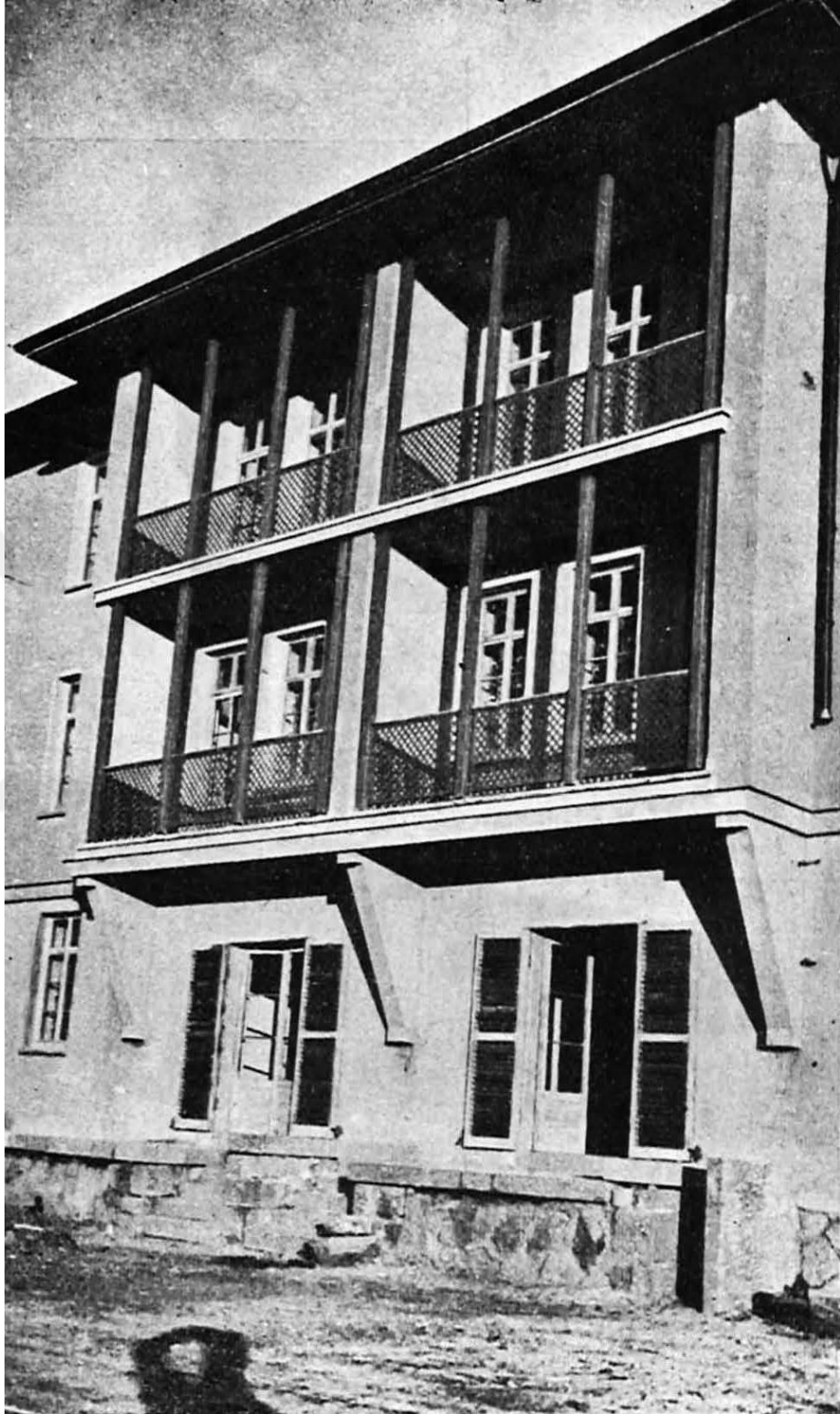
Figure 2.12: One of the housing facade of Saraçoğlu Neighborhood (Type B) (Sayar, 1946).
