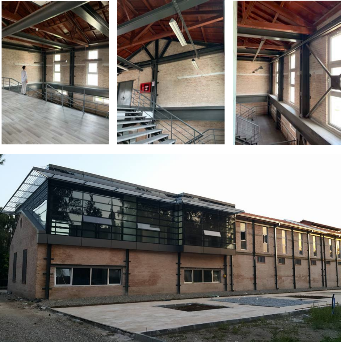
Figure 4.58: Inside and Outside of the Museum Complex Office Building ( 2019, Çağlayan, S. and 2016, M. Şekercioglu Archive)
