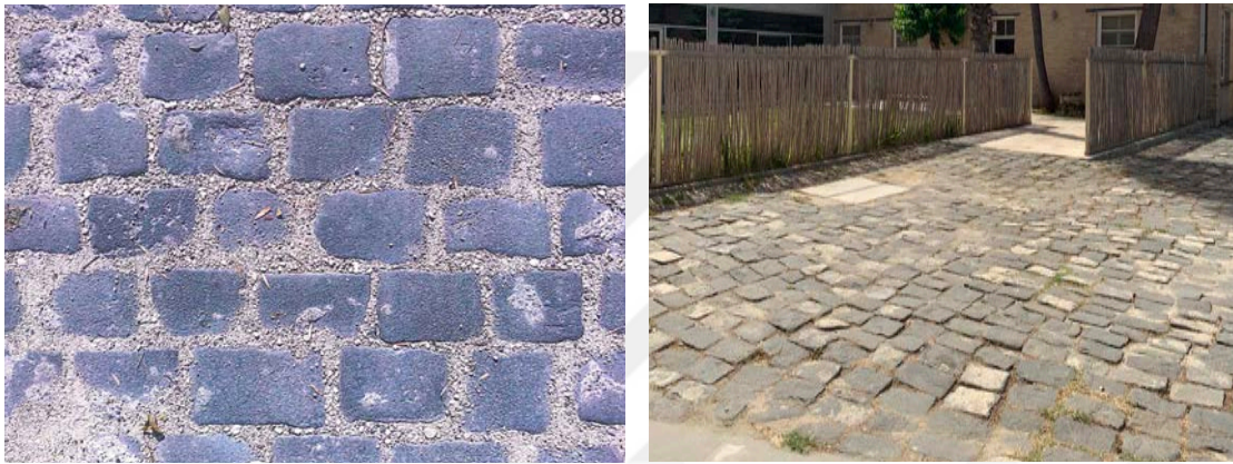
Figure 4.40: Basalt stone parquet flooring ( 2013 and 2019, Adana Directorate of Surveying Monuments archive by Miyar Architecture and Çağlayan, S.)
