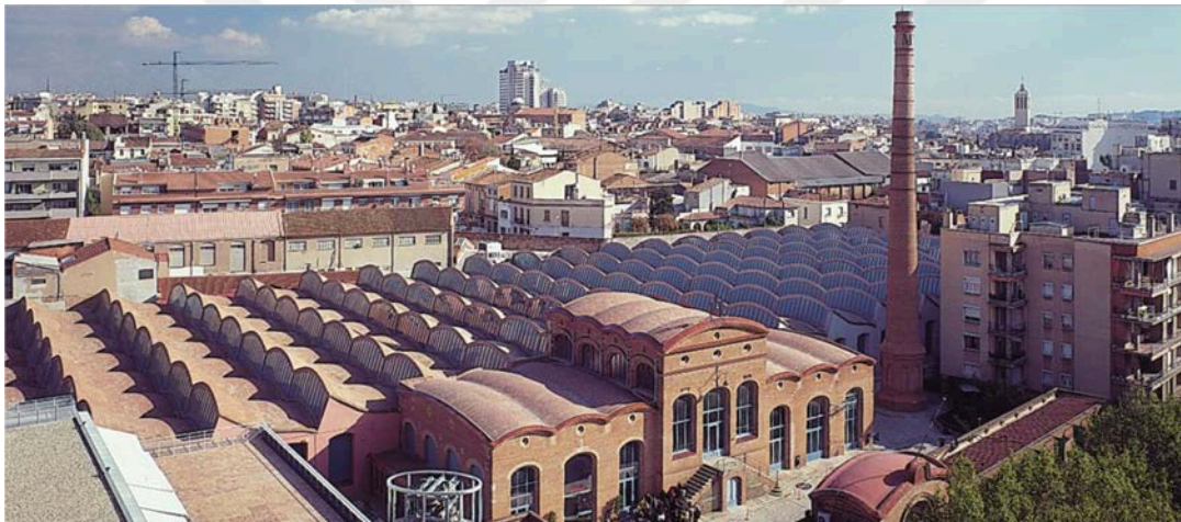
Figures 3.4. National Museum of Science and Industry of Catalonia/ The Photo showing its Situation after Conservation (1995, Url 7)
