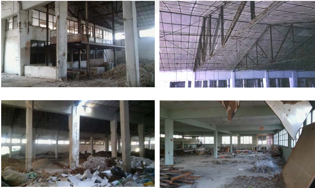
Figure 4.65: Interior of Spining Mill Building ( 2016, K. Celayir Archive)
