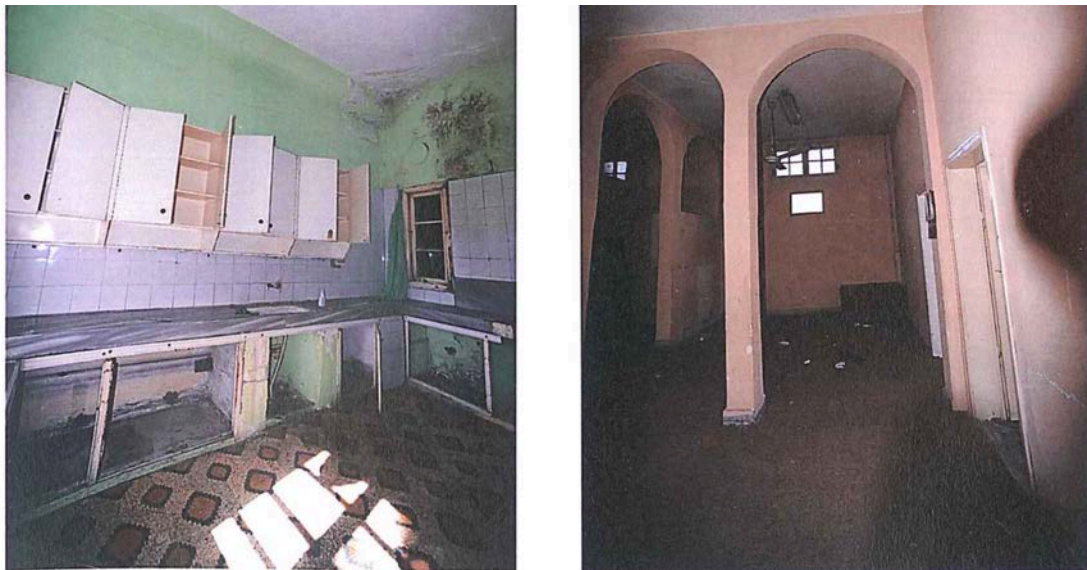
Figure 4.75: Interior of Local Building ( 2014, Adana Directorate of Surveying Monuments Archive by Miyar Architecture)
