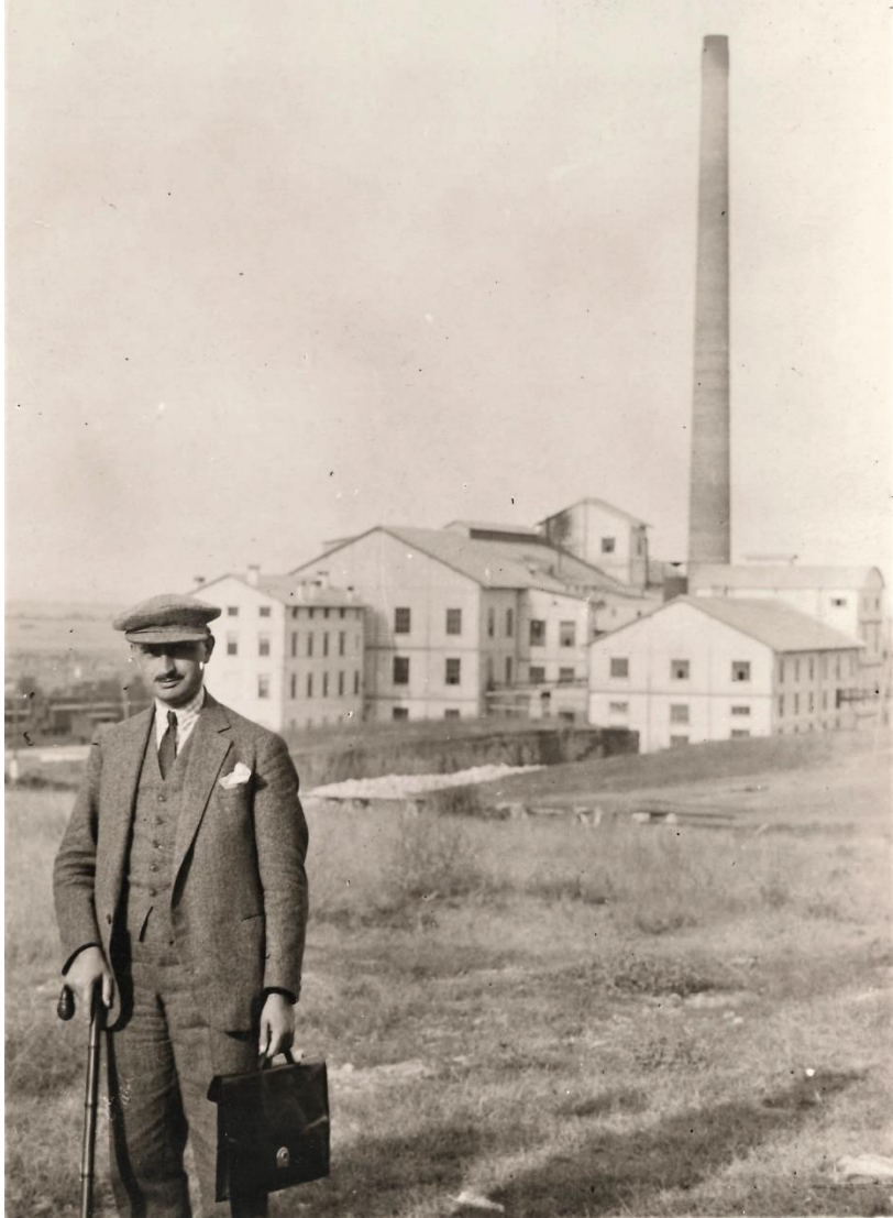
Figure 2. 3: Alpullu Sugar Factory (TOBB ETU Architecture Department Archive).
