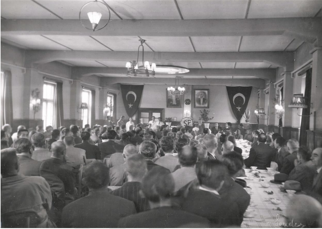
Figure 2. 17: Eskişehir Sugar Factory, Assembly Hall (TOBB ETU Architecture Department Archive).
