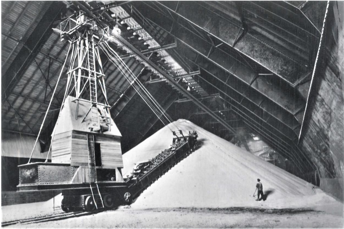
Figure 2. 2: Alpullu Sugar Factory (TOBB ETU Architecture Department Archive).
