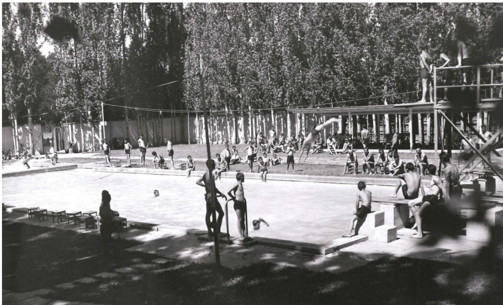
Figure 2. 14: Turhal Sugar Factory, Swimming Pool (TOBB ETU Architecture Department Archive).
