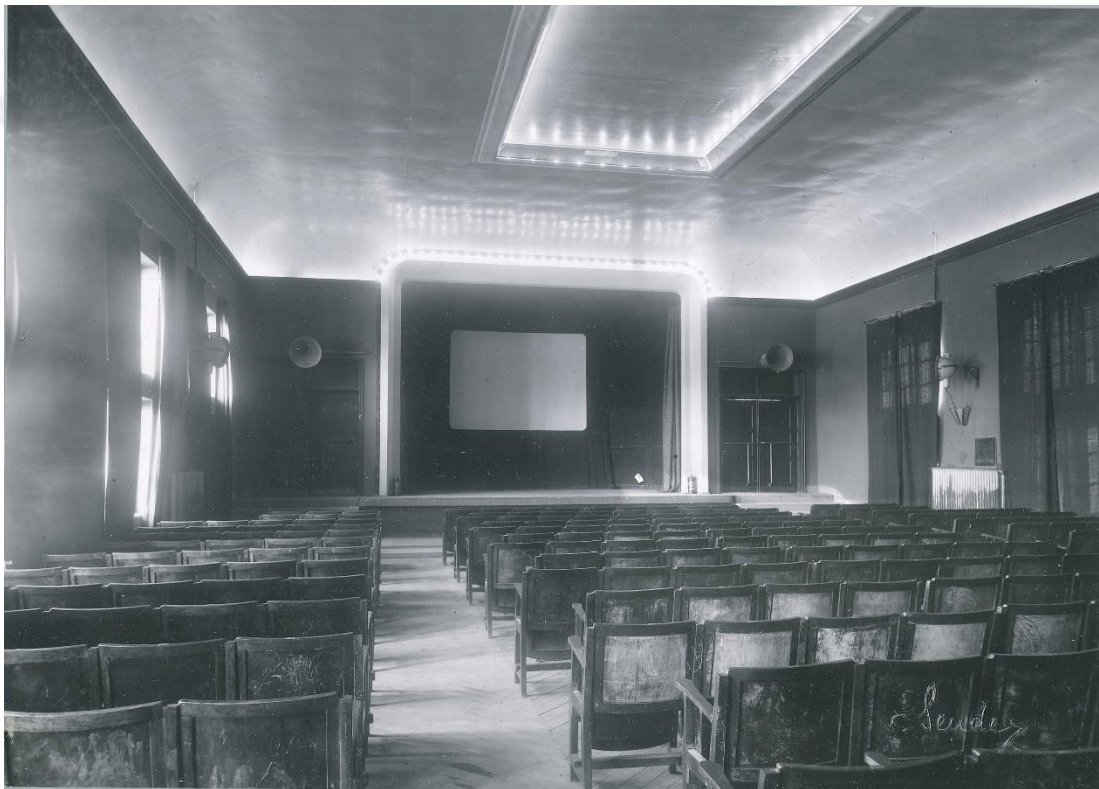
Figure 2. 12: Turhal Sugar Factory, Cinema Hall (TOBB ETU Architecture Department Archive).
