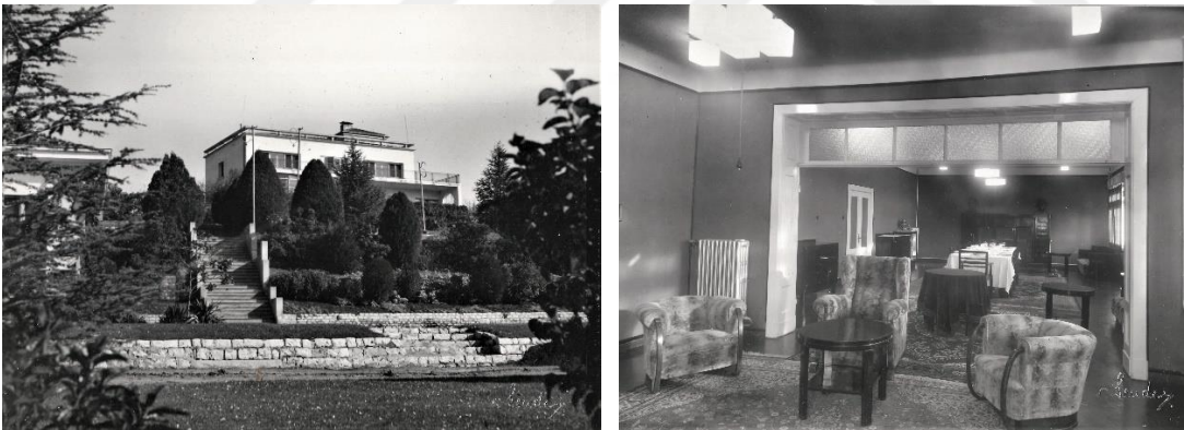
Figure 2 18: Ergene Villa Guesthouse (TOBB ETU Architecture Department Archive).
