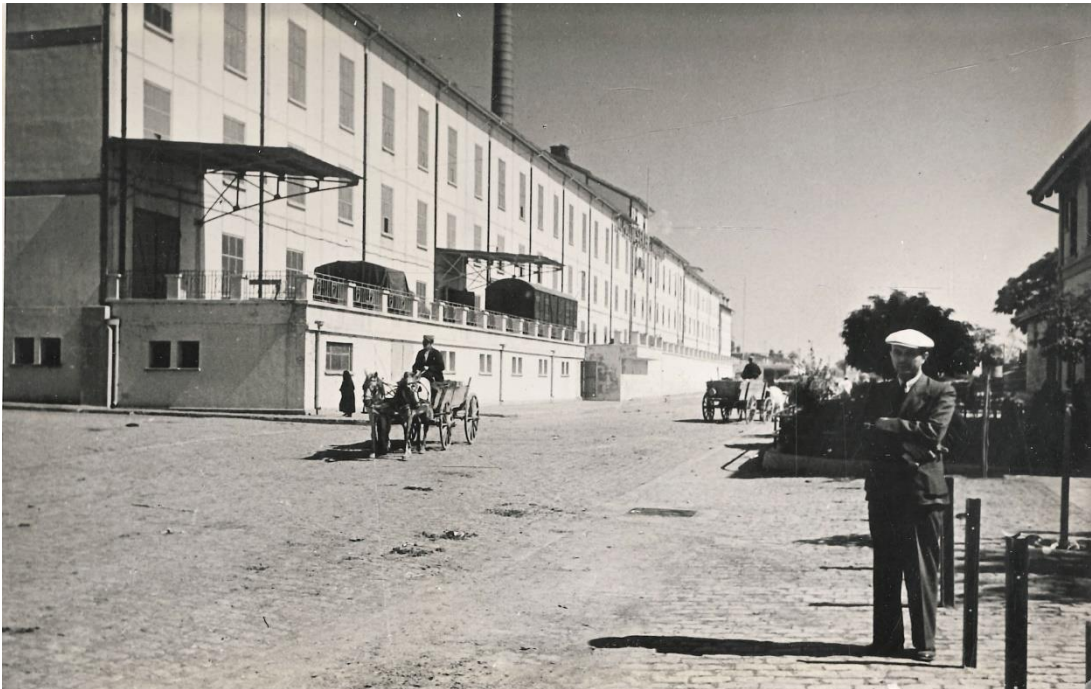
Figure 2. 4: Alpullu Sugar Factory (TOBB ETU Architecture Department Archive).
